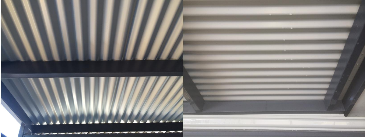
(Pictures of the same areas of patios after simple cleaning with a scourer and water)
